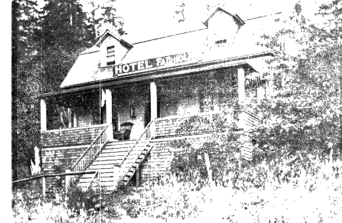
Fairholm Resort in its early days - Fairholm Resort in 1916 on Lake Crescent, owned and operated by Capt. Home and was later sold to Al Fairservice. Many changes have taken place since that time. Complete story and picture story on pages 4 and 5.
